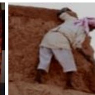
FIGURE 38. Cob (labin) construction
