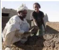
FIGURE 21. Cob as a building material used in buildings by house owners
