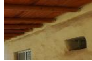
FIGURE 22. Cob's timber roofing sheet
