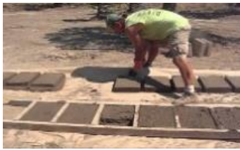
FIGURE 12. multi-framed to produce a large number of blocks in limited time
