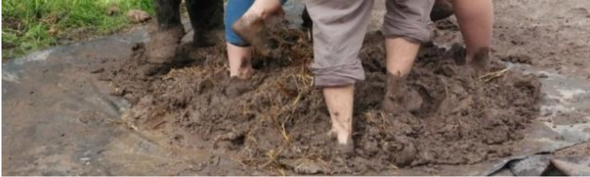
FIGURE 15. Adobe prepared by mixing the soil, which often contains a high percentage of silt or clay with water with the addition of hay or chopped straw or other plant fibers, then well mixed by foot or using the bulls or cows dung
