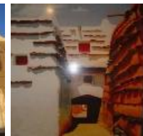
FIGURE 37. Projecting course of flat coral stones technique
