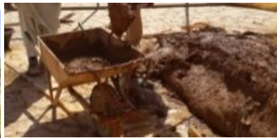
FIGURE 41. The mixing up process by The mixers (mulabineen) feet
